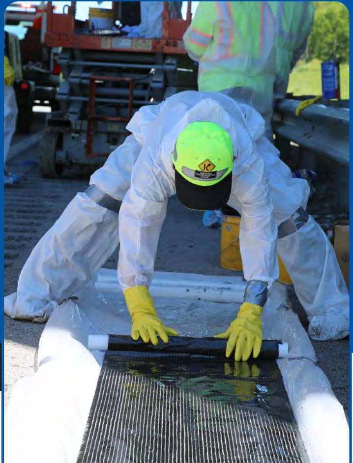
CatStrong products are designed for faster and more efficient application, reducing labor hours and equipment costs that are typically necessary for bridge maintenance projects.
