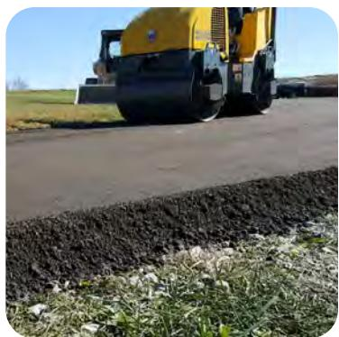
asphalt (HMA) overlay, in-place recycling and reclamation of asphalt pavements is rarely practiced in Kentucky and is not a well-defined process. It is widely known that when pavement sections become too deteriorated, in-place recycling and FDR preservation techniques do not produce good results.
