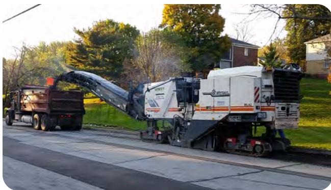
A second preservation technique, in-place pavement recycling, takes the degraded top layer of pavement and restores the roadway to an even surface. Both methods require a new hot mix asphalt (HMA) layer over the stabilized layer, followed by shaping and compaction.
