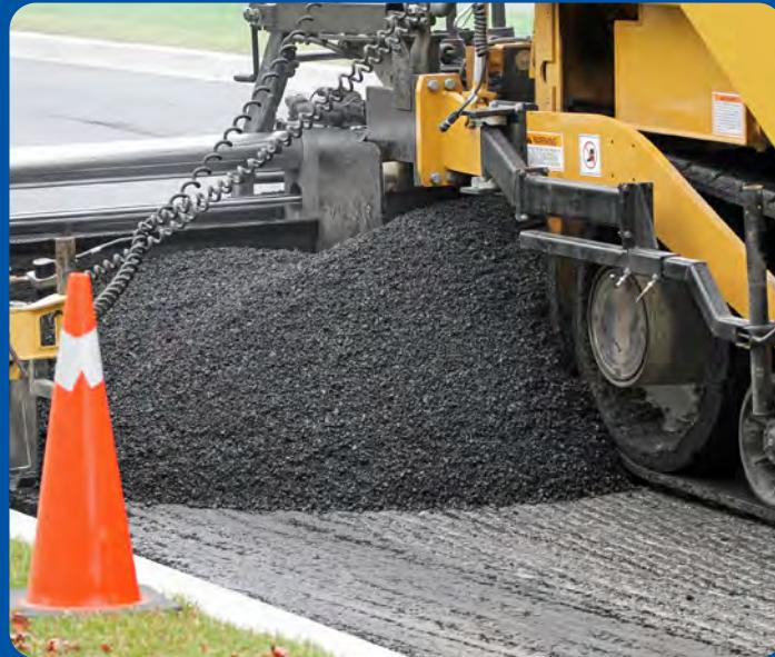
FDR can rehabilitate worn asphalt pavements while maintaining pavement geometrics and layer thicknesses. Furthermore, FDR conserves energy and natural resources and is an ideal solution for rehabilitating routes with low traffic volumes on which multiple base failures have occurred. Researchers also suggested creating a program focused on quality control/quality assurance testing and monitoring to verify design performance.
